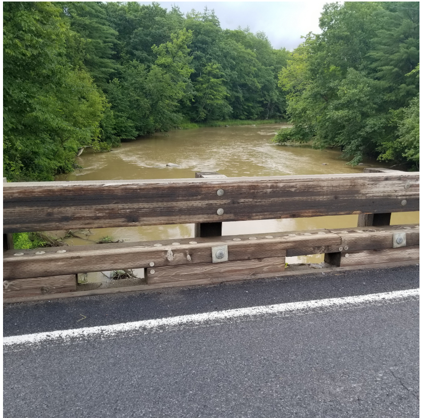
Photo 1: The Boquet River at Morehouse bridge.
