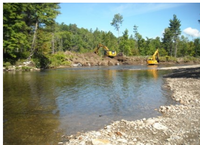
Working on the toewood structure
