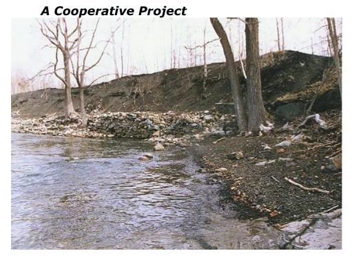
The two-tiered log cribbing structure, stretching 150 feet along the salmon pool below Willsboro falls, has been completed by Moriah Shock inmates under the supervision of John Northup, ENCON Supervisor. Work was hard and dirty due to a 35-foot tall embankment of loose black ash residue from the former pulp mill, upstream ledge rock, and downstream timbers and concrete. Nevertheless, John Northup once again illustrated his skill at turning BRASS designs into reality.
