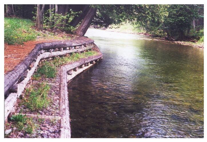
Photo taken during the summer. Note how far the angled section of the crib has slumped down into the water. The large hemlock tree in the background had listed before the crib was constructed, but with the slump it looks even more precarious.
