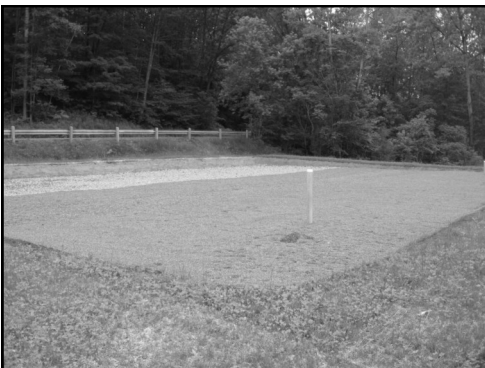
The pretreatment cell, which will be planted with wetland vegetation.
