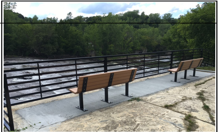
New Benches and Railing provide a beautiful viewing area located over the old fish ladder. Photo courtesy Jeff Clock, August 2016
