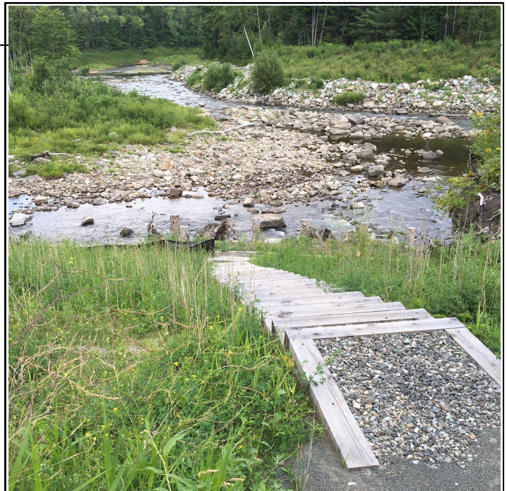
New Fishermen Stairway Photo courtesy Jeff Clock, August 2016
